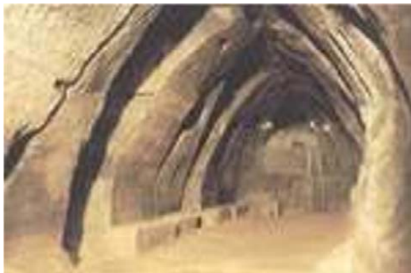
ice storage cave in Bliesdahlheim
